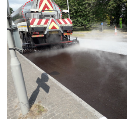
Road investment – highway maintenance in BCP.
