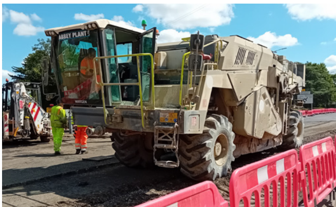
Using recycled materials to reduce the carbon footprint of construction – works on the A341 on Wimborne Road in BCP.
